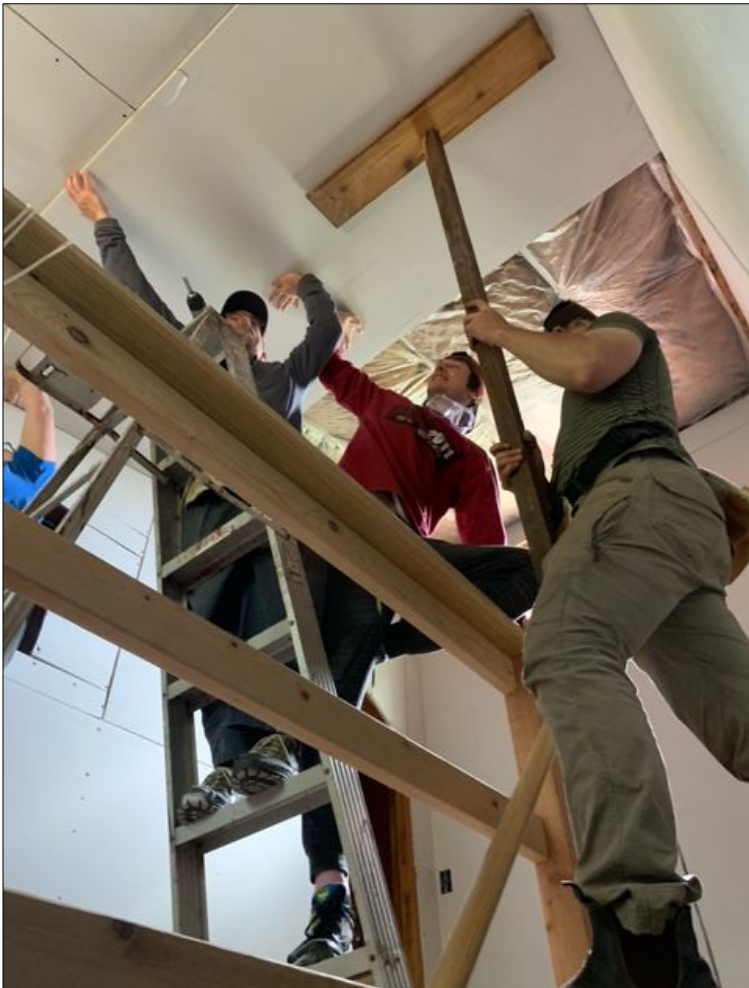
Renovating the new home of Benincasa Community, CT (photo © Benincasa Community)
